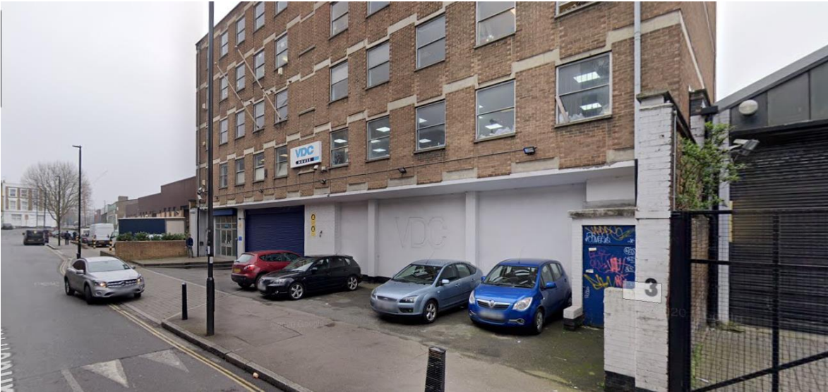
Fig. 10.10: Front of existing Site
