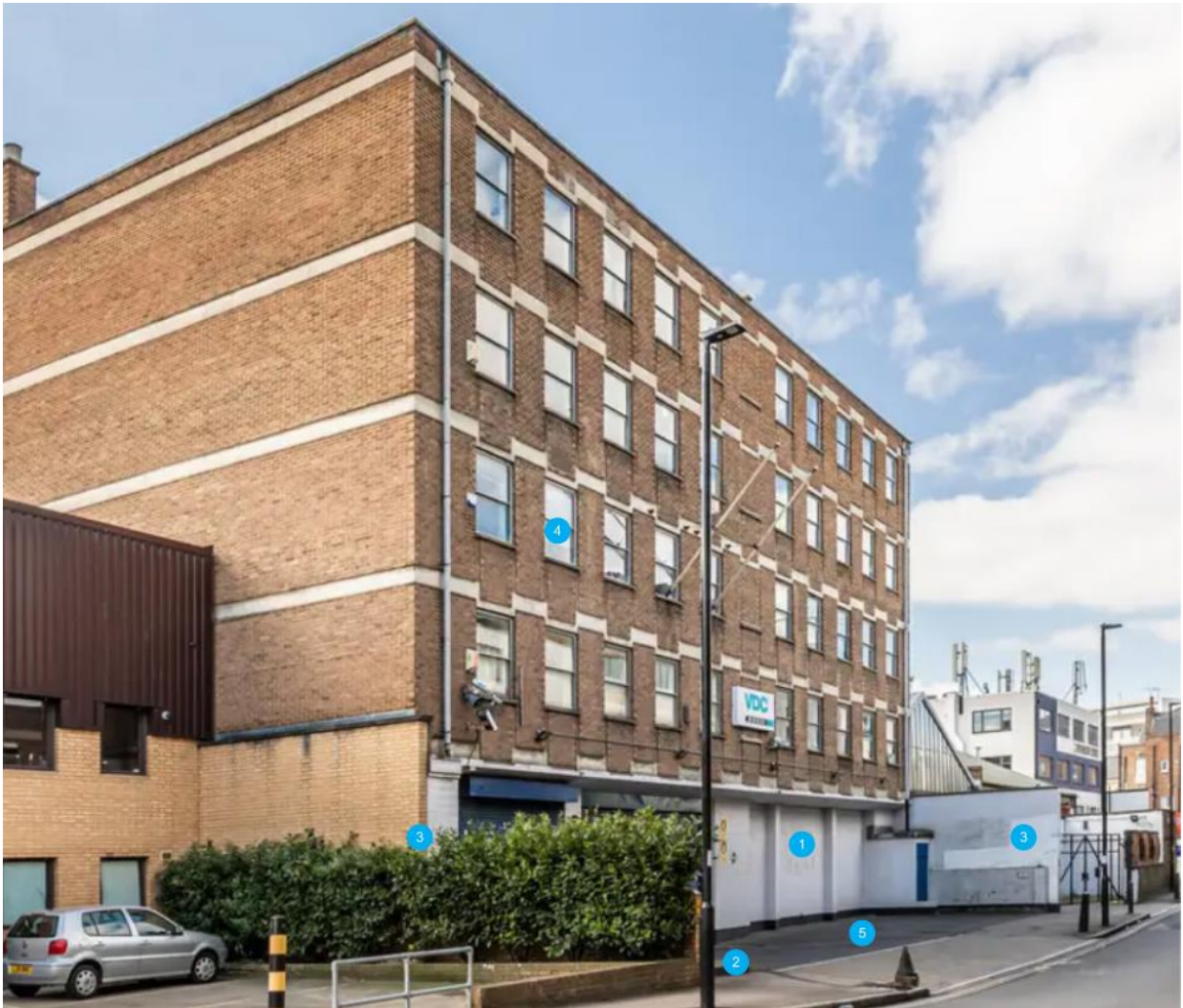
Image 3.3: View of building's front / street elevation looking west along Brandon Road
